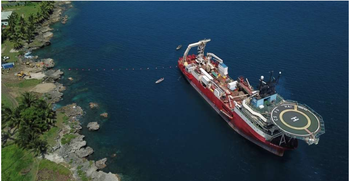
Figure 1: PNG Data Co. installing a fibre optic cable, off the coast of Papua New Guinea (source: https://www.pngdataco.com/ )
